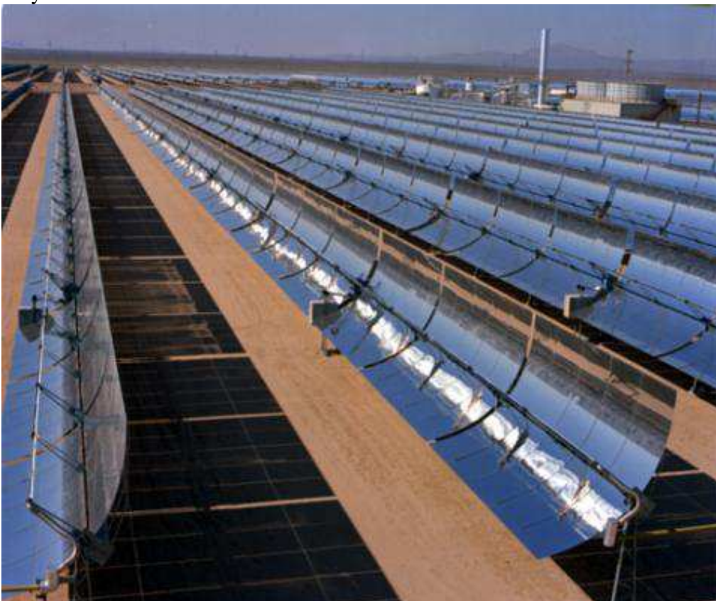
30. ábra. Napvályús naperőmű NextEra Energy Resource's Bakersfield power plant http://www.heatingoil.com/blog/water-hindering-renewable-energy-projects106/
